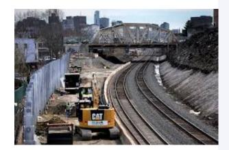
Construction began on an ambitious Green Line Extension project in January 2020. This project entails the rehabilitation and replacement of track on the concrete arched structure across from the Science Museum to accommodate heavier loads and increased train frequency, while preserving the viaduct's historic façade. Read more **here**
